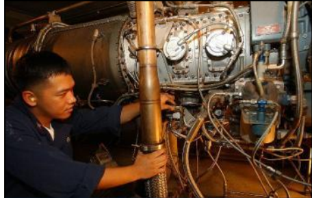
Allison 501k G/T Generator January 2011
